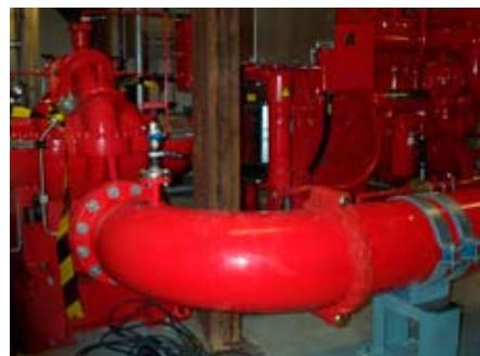
Alvenius® Thermoplastic Coated pipes are used in the fire protecting system at Ringhals nuclear power plant, Sweden.
